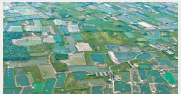
養殖輸水工程 Water Supply engineering
