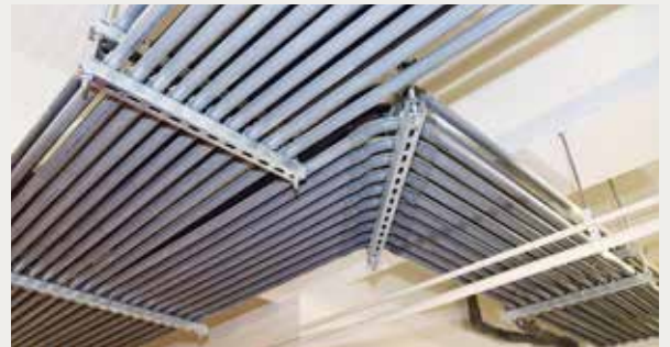
建築工程 Architectural engineering
